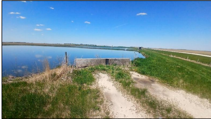
Figure 4 Cell 1 septage dump
